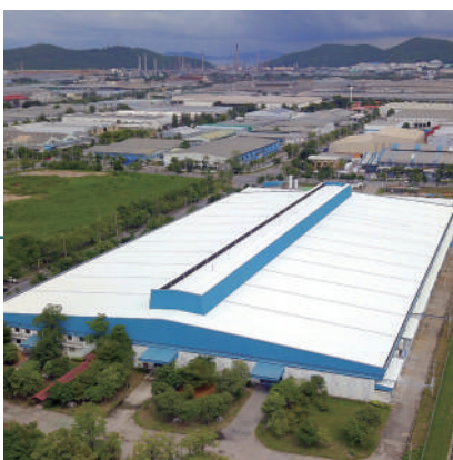
Fujitsu General (Thailand) Co., Ltd. (Thailand) Factory-2
